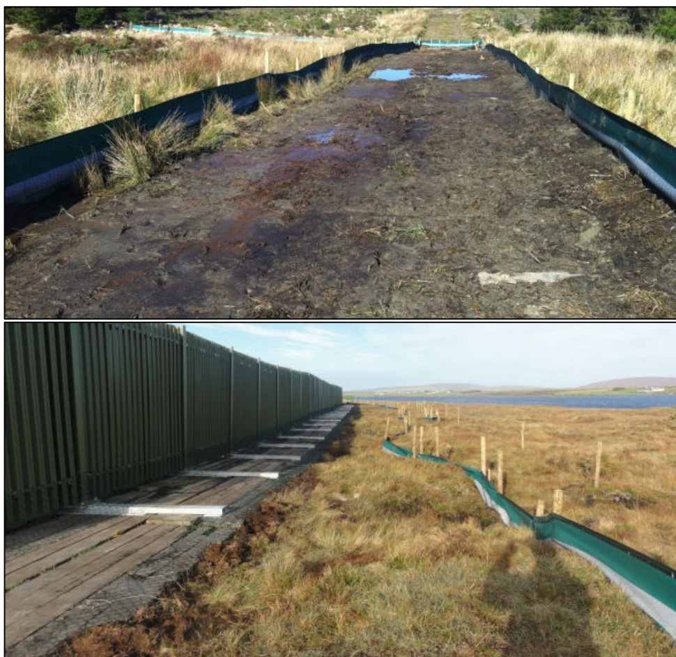
Plate 2-4 Typical Silt Fence Details
