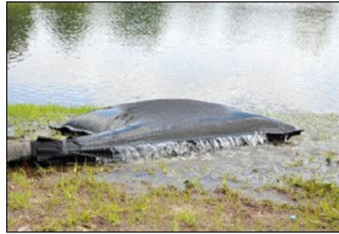
Plate 2-2 Silt Bag with water being pumped through
