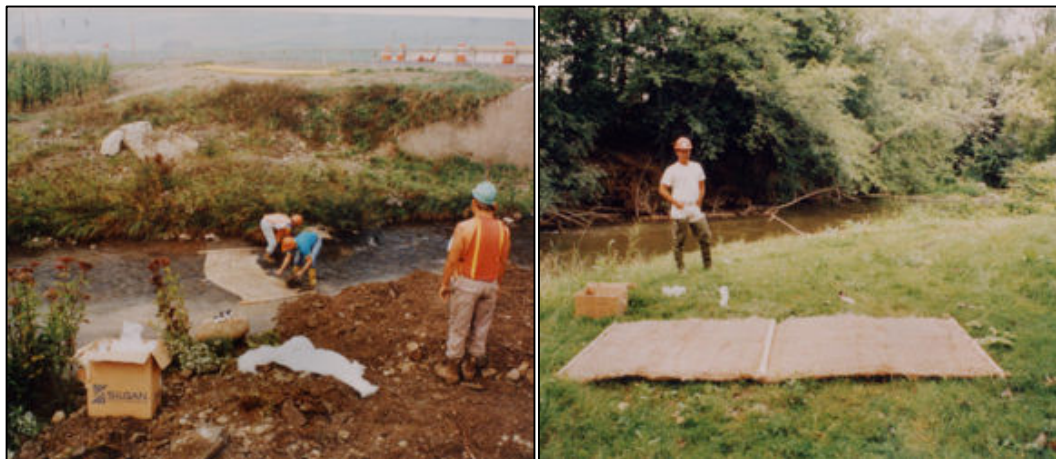
Plate 2-3 Typical Sedimat Details (Source: https://www.hy-tex.co.uk/ )
